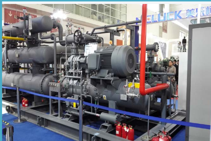
System - AIST modular unit (cascade room)
